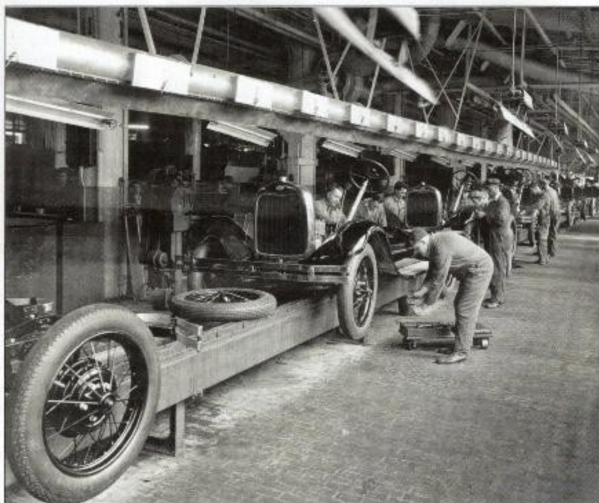
Rouge Plant, Dearborn, Michigan, April 10, 1928.
